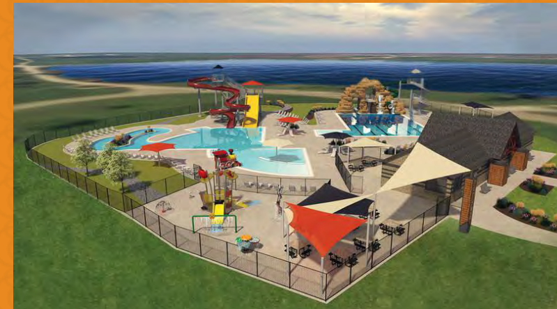
McKinley Park Aquatic Center – Creston
